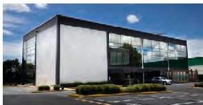
302 Great South Road, Greenlane
