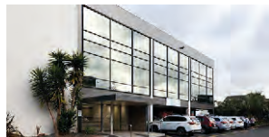
308 Great South Road, Greenlane
