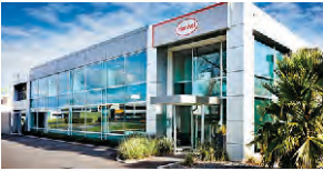
106 Springs Road, East Tamaki
