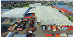
240 Puhinui Road, Manukau
