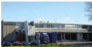
80 Springs Road, East Tamaki
