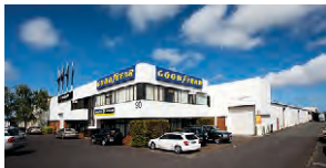
90 - 104 Springs Road, East Tamaki
