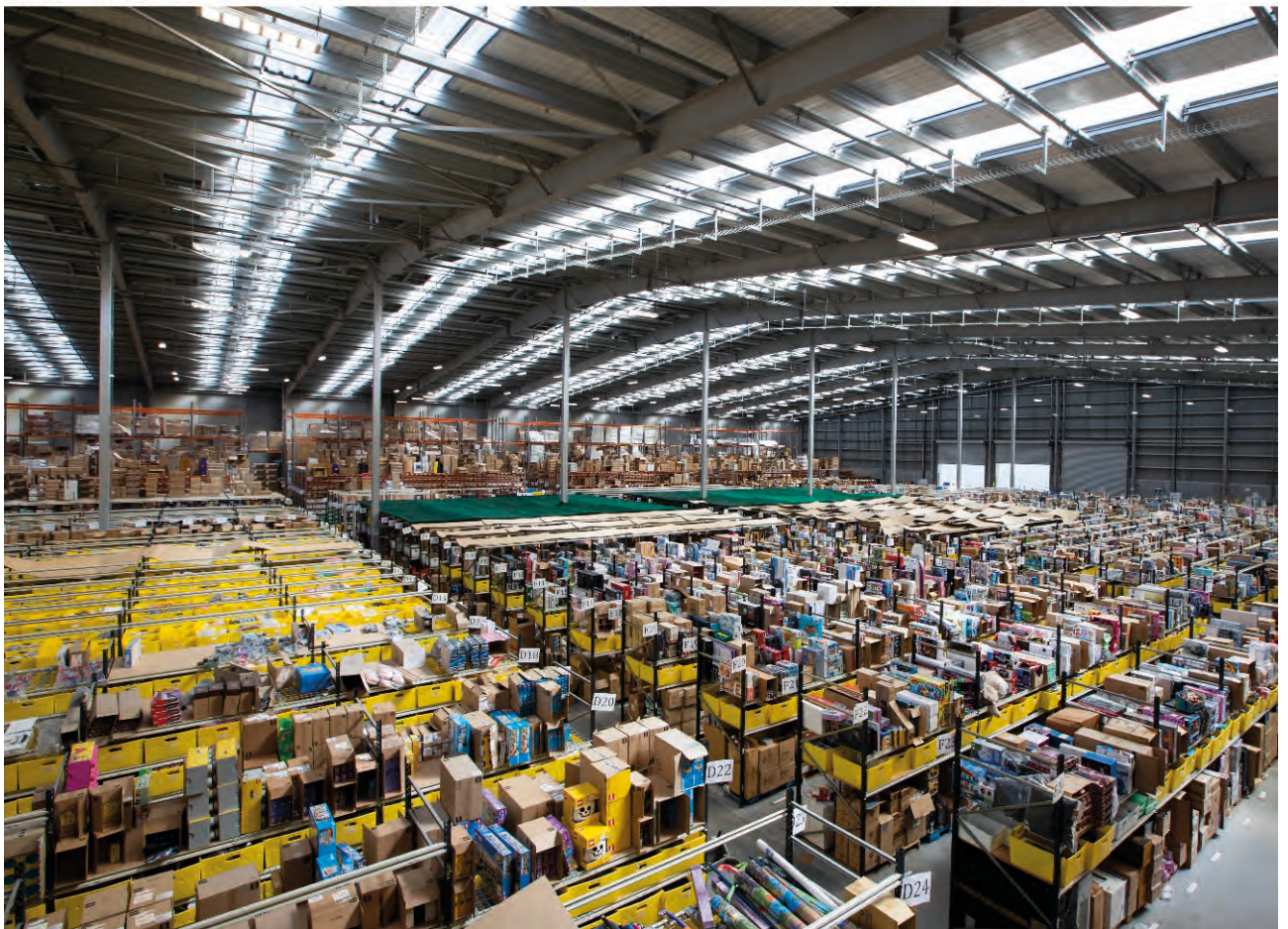
Highgate Parkway, Silverdale, Mighty Ape Head Office / Distribution Warehouse
