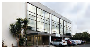
308 Great South Road, Greenlane
