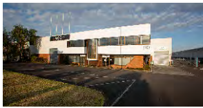
90-104 Springs Road, East Tamaki
