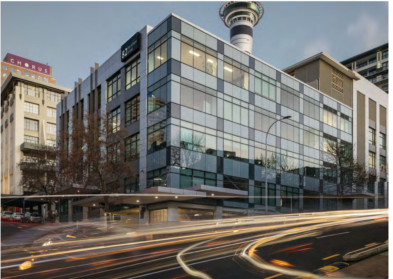
Bottom: 82 Wyndham Street, Auckland
